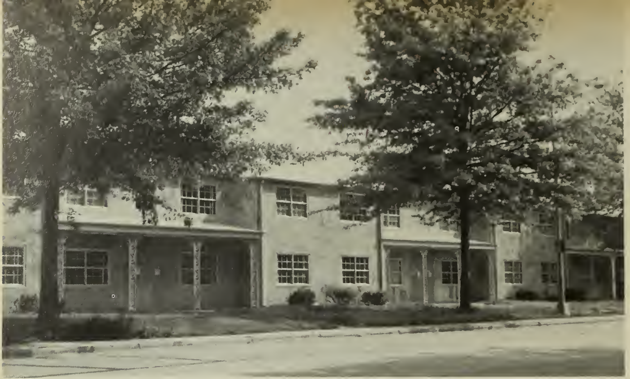
NEW LOOK—Benmoreel Navy Housing in Norfolk, Va., is being renovated.
